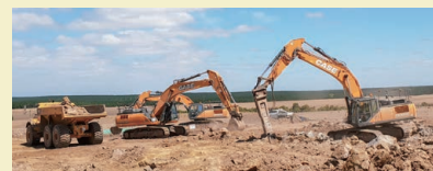
KANAMOTO AUSTRALIA HOLDINGS PTY LTD
