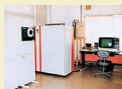
Computer Division equipment room in the 1980s
