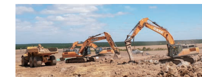
KANAMOTO AUSTRALIA HOLDINGS PTY LTD
