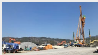
岩手県下閉伊郡山田町の地盤改良工事 Yamada-cho Ground Improvement Work in Shimohei, Iwate
