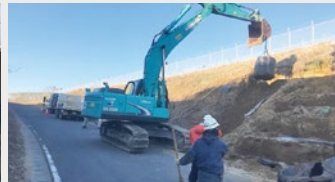
千葉県成田市の空港法面復旧工事 Airport Slope Restoration in Narita City, Chiba
