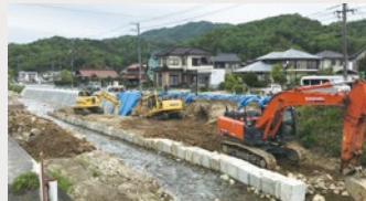
広島市安芸区の瀬野川災害復旧工事 Seno River Post-Flood Reconstruction in Aki Ward in Hiroshima City
