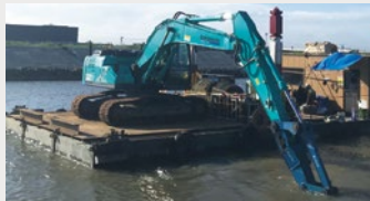
宮城県岩沼市の五間堀河川災害復旧工事 Gogenbori River Post-Flood Reconstruction in Iwanuma City, Miyagi
