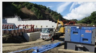
北海道勇払郡厚真町のメナノ沢川災害関連緊急砂防工事 Emergency Menano-sawa River Construction to Prevent Erosion in Atsuma, Yufutsu in Hokkaido
