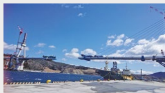
宮城県気仙沼市の気仙沼湾横断橋工事 Kesennuma Bay Bridge Construction in Kesennuma City, Miyagi
